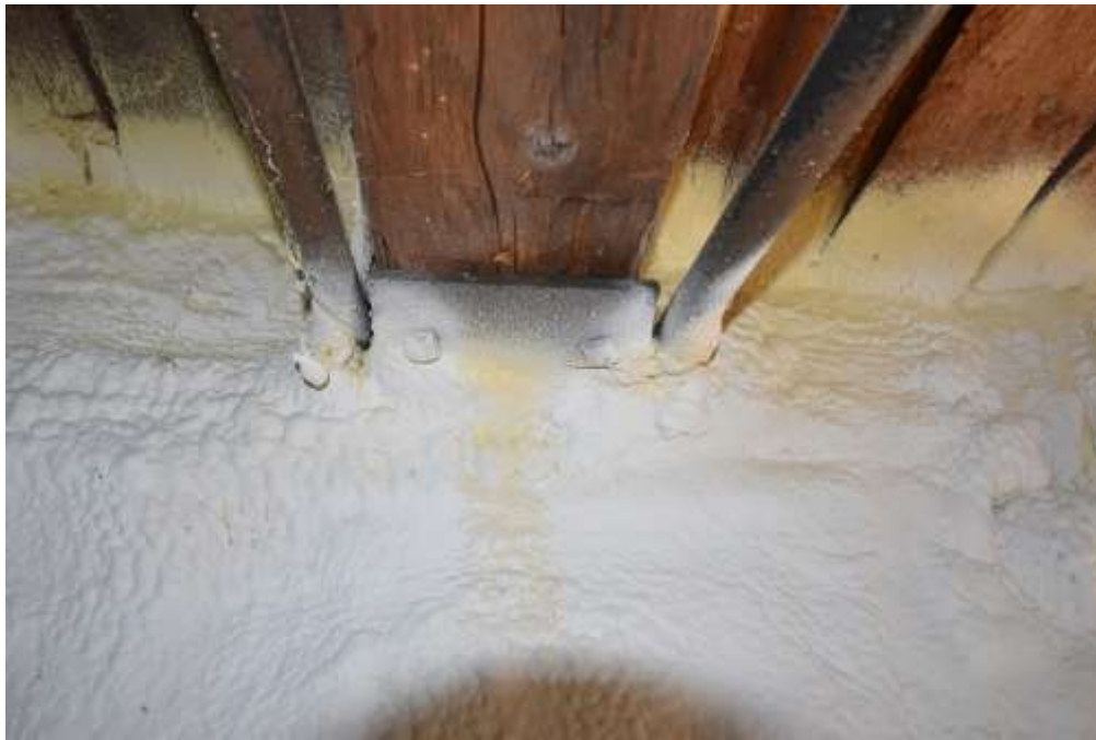
Figure 1, Floor Truss Tie Rod Connection
